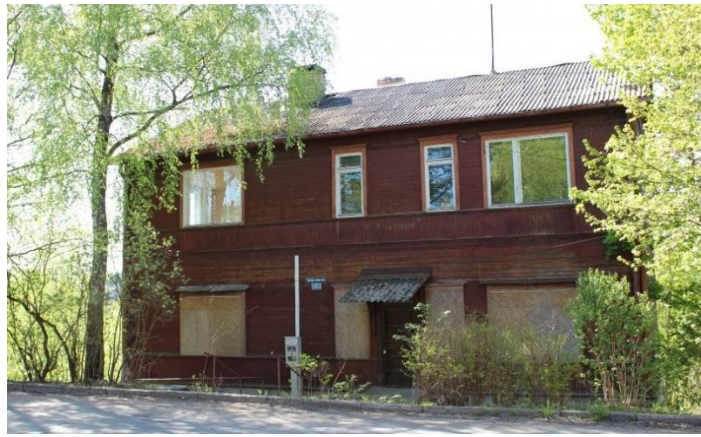
Picture 1 The building of the Centre for Creative Ideas in Rezekne, Seiles street 1a, before reconstruction
